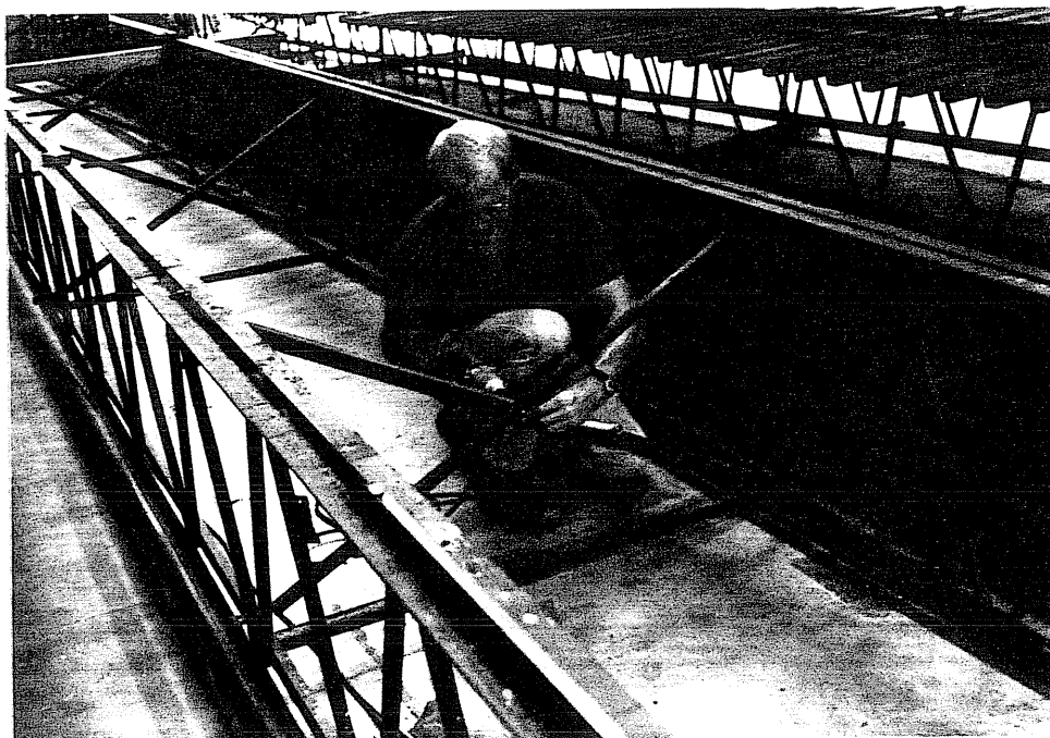
Figure 2.7 Photograph of Cross-Bracing Installation
